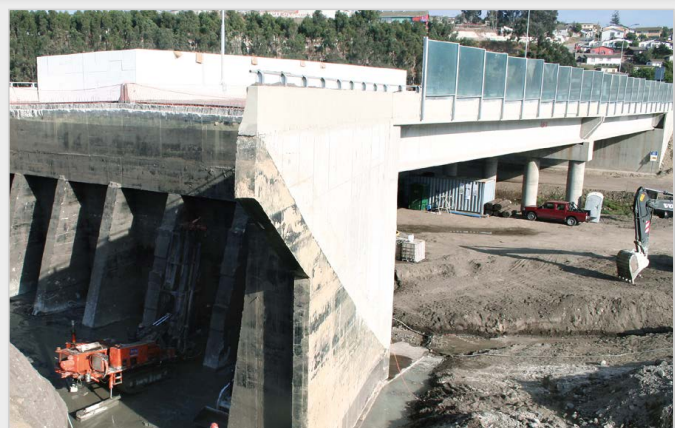
Bridge abutment underpinned in 2009 with 40 TITAN 103/78 micropiles in a region in Chile with high seismic activity.
