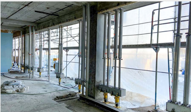
TITAN SLS aluminium heavy-duty props allow for precise adjustment of the required prestress
