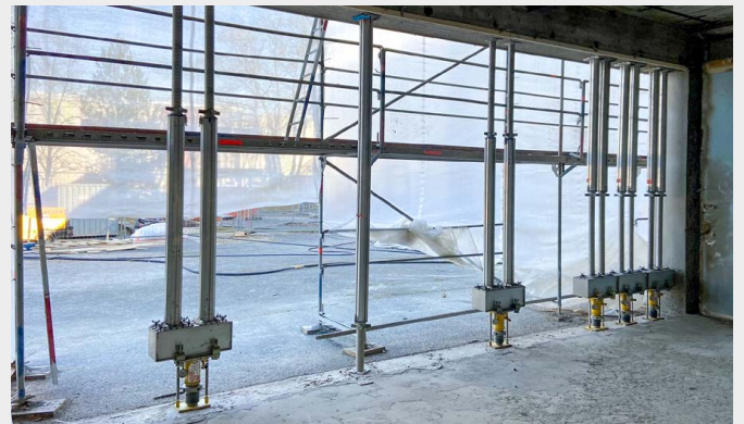
The props are raised and lowered manually with a lever on each hydraulic jack
