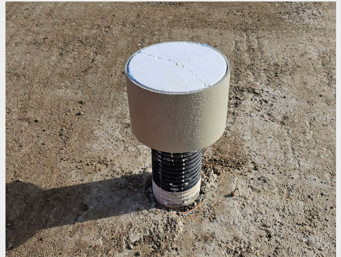
A polystyrene cap enabled the settlement of the foundation slab without transferring the compressive forces to the micropiles
