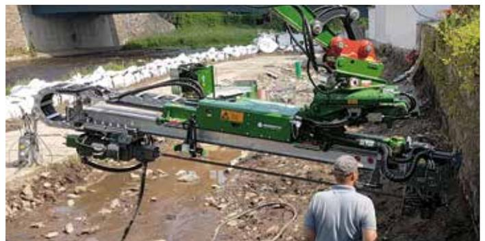
TITAN 30/11 micropiles were used to upgrade existing retaining walls.
