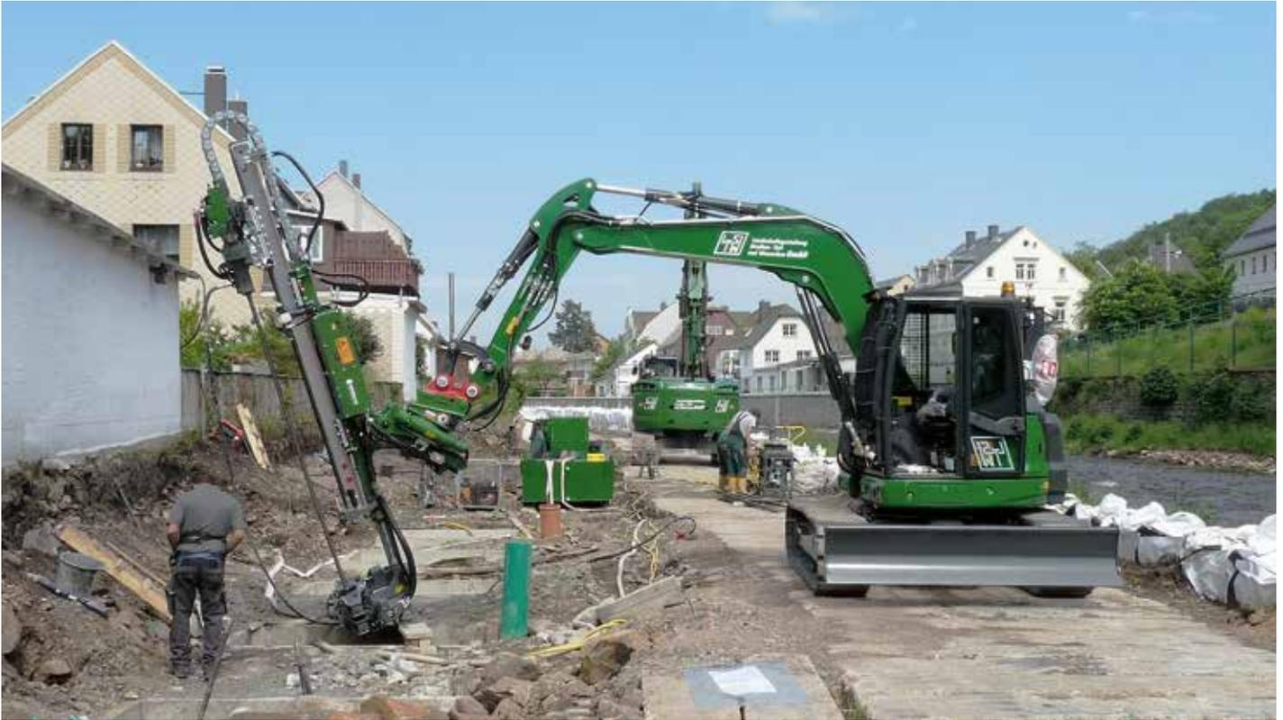
Ischebeck TITAN 40/16 and TITAN 52/26 micropiles were used in the foundations for new retaining walls in this section of the flood defences.
