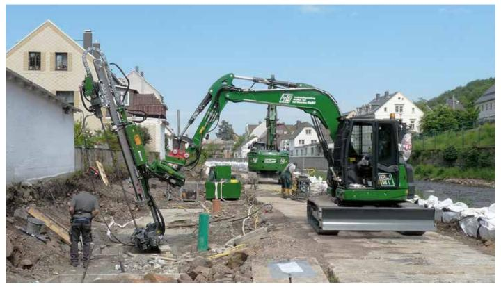
Ischebeck TITAN 40/16 and TITAN 52/26 micropiles were used in the foundations for new retaining walls in this section of the flood defences.
