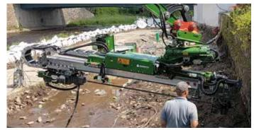
TITAN 30/11 micropiles were used to upgrade existing retaining walls.
