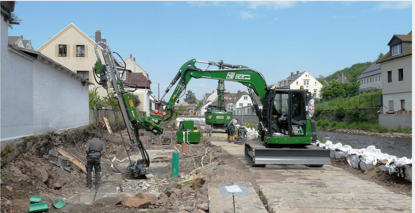
Ischebeck TITAN 40/16 and TITAN 52/26 micropiles were used in the foundations for new retaining walls in this section of the flood defences
