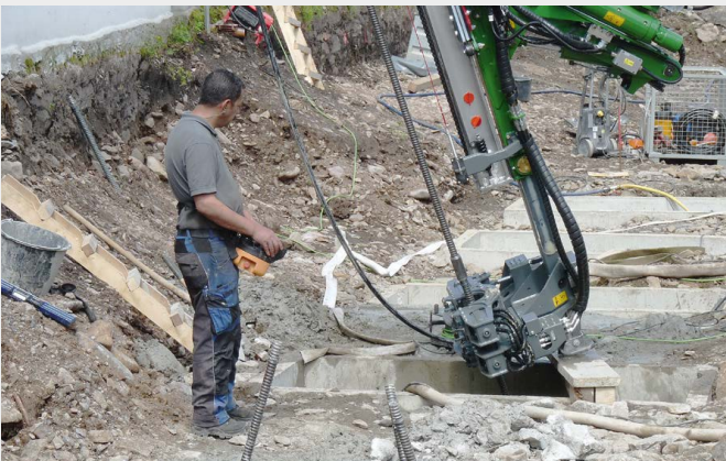
TITAN micropiles are approved for permanent applications (100+ years, DIBt approval Z-34.14-209)
