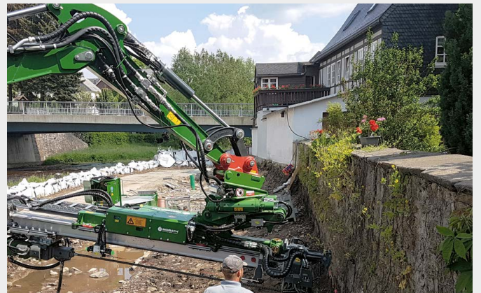
TITAN 30/11 micropiles were used to upgrade existing retaining walls
