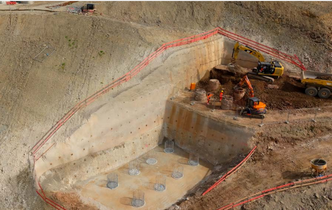
Shotcrete walls anchored with TITAN micropiles, protect the excavation pits for the bridge piers
