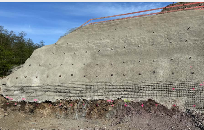
TITAN micropiles and steel mesh with shotcrete
