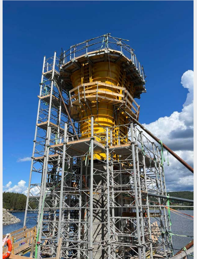
Megashore stair case, column formwork and steel BKS push and pull props
