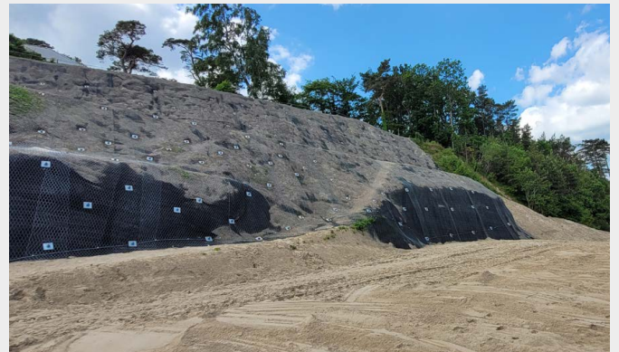
The soil nails were used in combination with a steel net and an erosion control mesh
