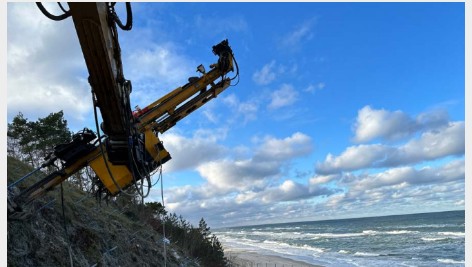
Despite the challenging slope at the site, it was possible to install the soil nails with small plant
