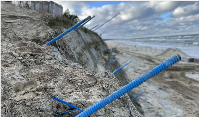
TITAN 40/27 micropiles as soil nails at an angle of 30°
