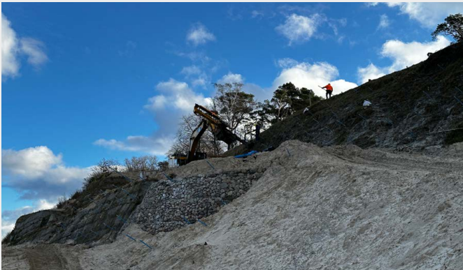
Stabilisation of the steep slope with TITAN micropiles as soil nails
