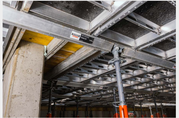
The TITAN HV aluminium slab forming system adapts flexibly to obstacles such as pillars
