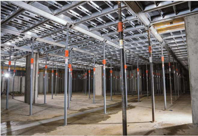
View of the TITAN HV aluminium slab forming system with TITAN HV 150 combi panels installed from below
