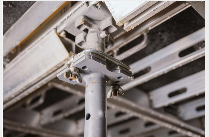
The drophead system allows early removal without relieving the props
