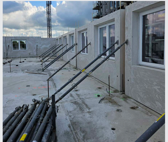
Use of the push-pull props as a thread element. All TITAN push-pull props have high tensile and compressive strength
