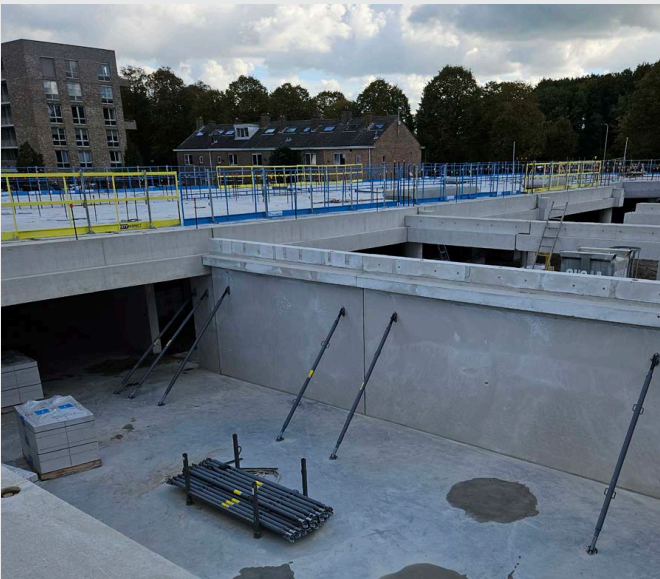
Overview of the precast walls in the basement
