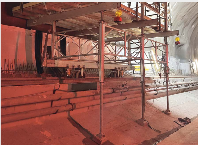
Swivel base plates were fitted underneath the TITAN adjustable legs to compensate for the angle of the base of the tunnel
