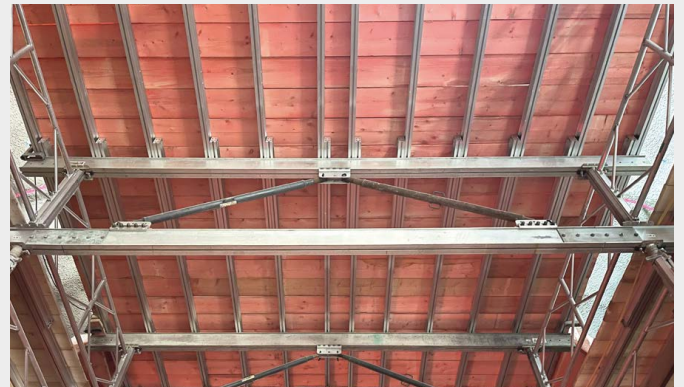
TITAN push-pull props distribute the horizontal loads acting on the topmost platform
