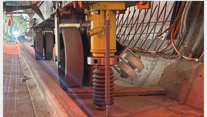
Fixed castors and hydraulic jacks were fitted to make the whole TITAN Megashore scaffold mobile
