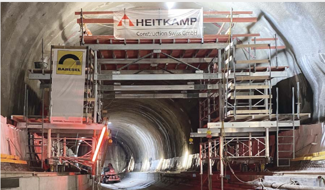
A mobile scaffold from Ischebeck was used to carry out work on the tunnel lining
