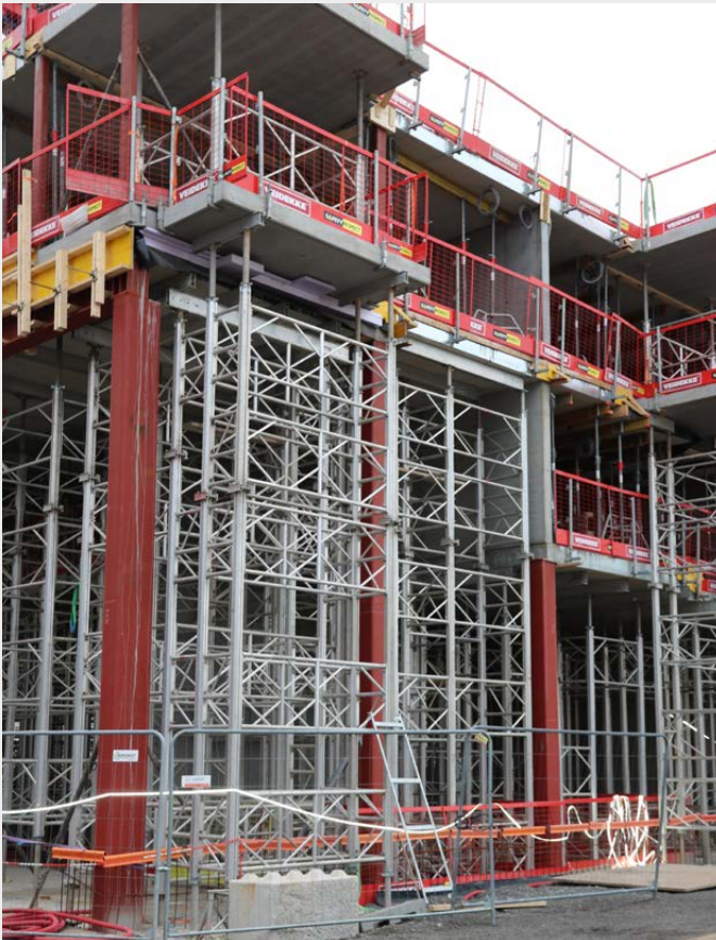
Megashore tower supports balconies for five levels, offering high capacity and stiffness
