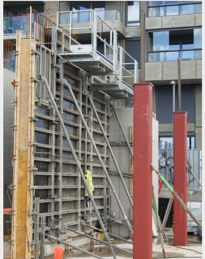
The picture shows Ischebeck TITAN RS push and pull props on a Noe wall panel
