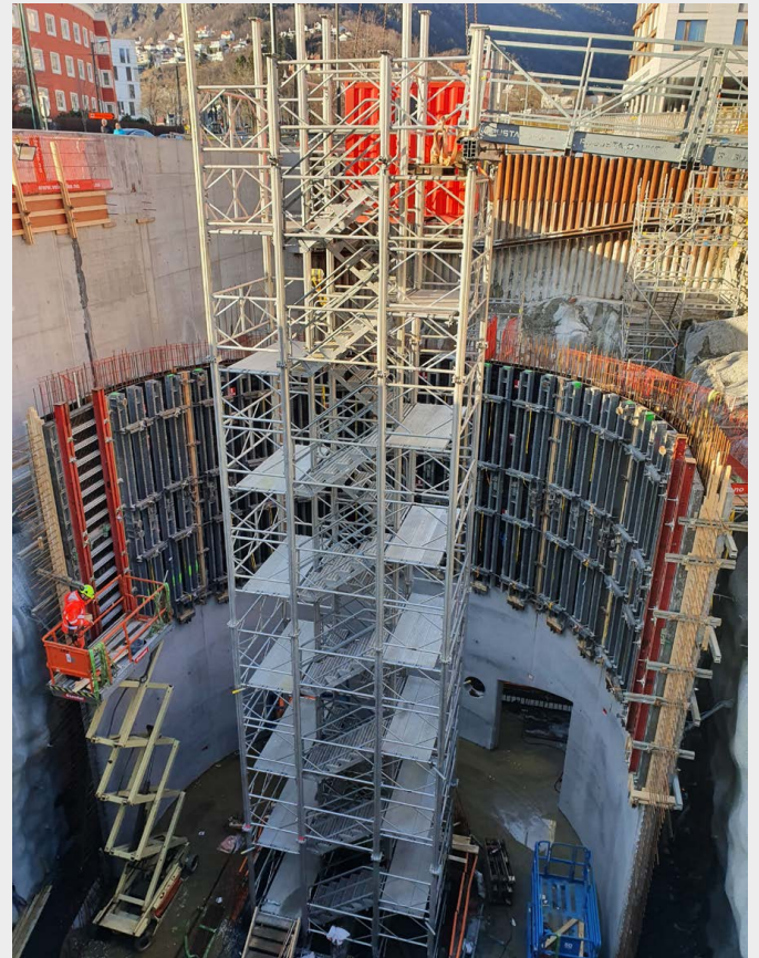
TITAN Megashore stair tower with Robusta-Gaukel Multi-Footbridge as a building site access
