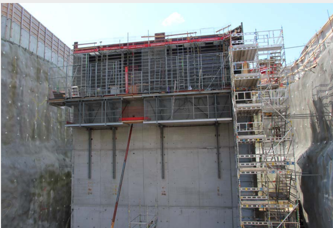
Boxer Climbtrac Auto, Hydraulic self-climbing system for high walls.
