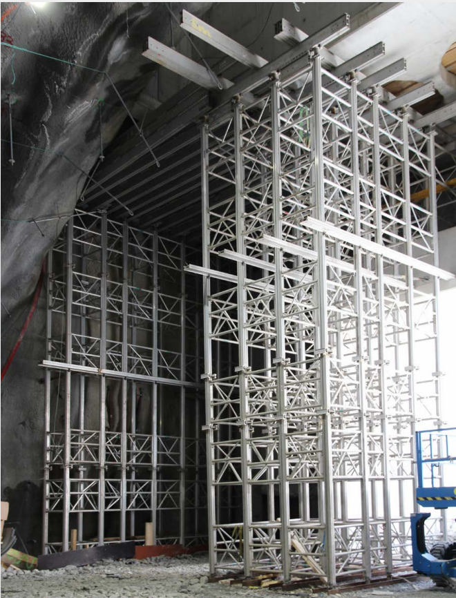
TITAN Megashore used to support the air ventilation shafts
