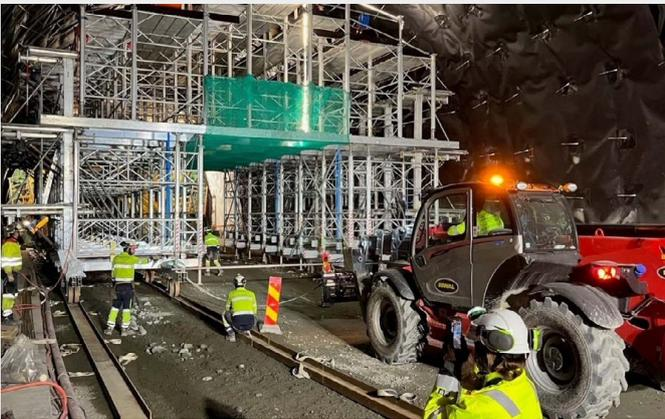
Horizontal repositioning of the tunnel wagon
