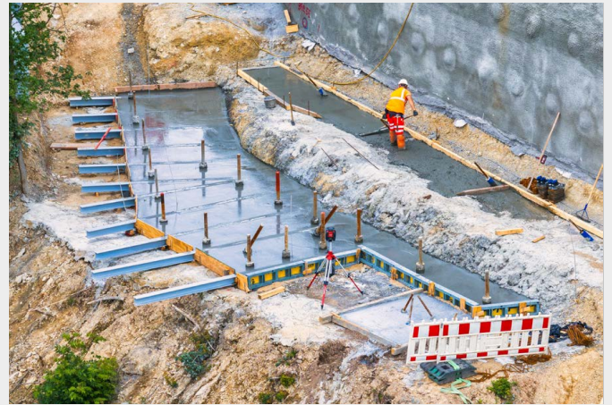
Shotcrete protection and foundations of the summit station
