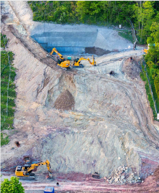
Excavation works at the valley station and shotcrete protection of the crane pad
