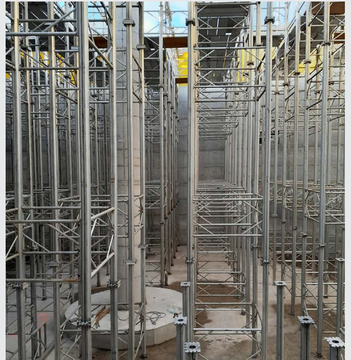
The TITAN Aluminium Megashore system is ideal for thick slabs due to its high load-bearing capacity
