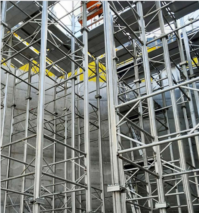
Passage decks with aluminium telescopic ladders enable quick and safe ascent
