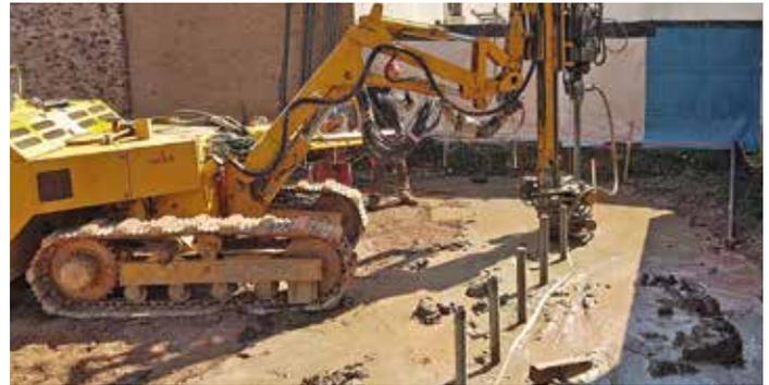
Self-drilling installation of micropiles on a confined site with a small drilling rig.
