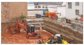
The first row of TITAN micropile anchors, with end plates already fitted.
