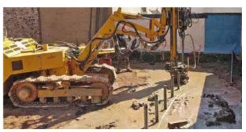
Self-drilling installation of micropiles on a confined site with a small drilling rig.
