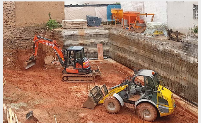
The first row of TITAN micropile anchors, with end plates already fitted
