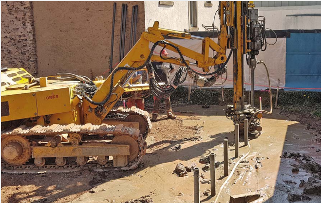
Self-drilling installation of micropiles on a confined site with a small drilling rig
