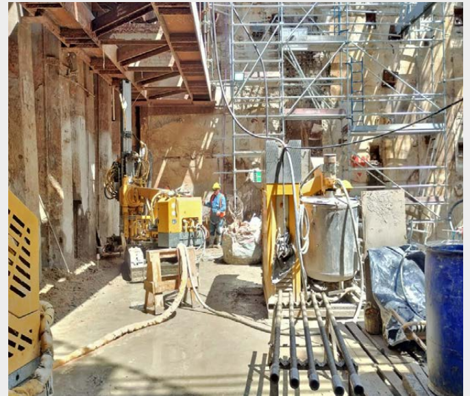
Confined drilling area, showing the drilling equipment in position and the pieces of a TITAN micropile ready to be installed
