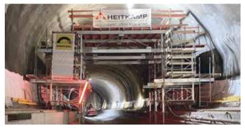
A mobile scaffold from Ischebeck was used to carry out work on the tunnel lining.
