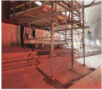
Swivel base plates were fitted underneath the TITAN adjustable legs to compensate for the angle of the base of the tunnel.
