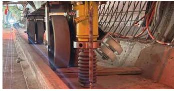
Fixed castors and hydraulic jacks were fitted to make the whole TITAN Megashore scaffold mobile.
