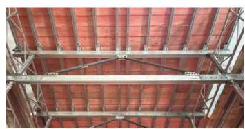
TITAN push-pull props distribute the horizontal loads acting on the topmost platform.
