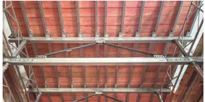
TITAN push-pull props distribute the horizontal loads acting on the topmost platform.
