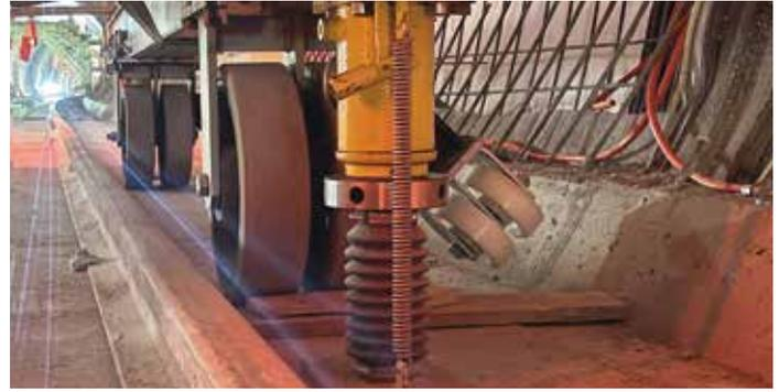
Fixed castors and hydraulic jacks were fitted to make the whole TITAN Megashore scaffold mobile.
