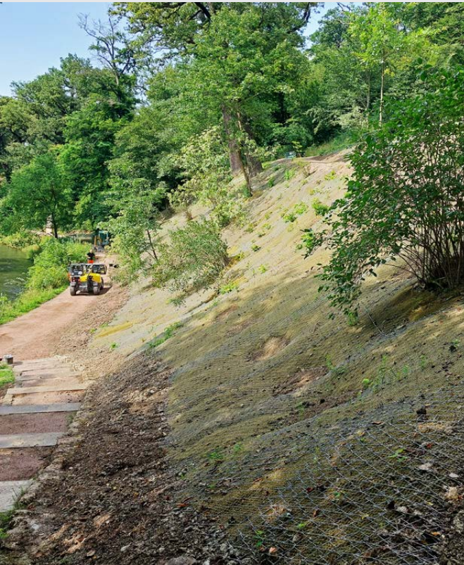
Completed slope stabilisation with vegetation already beginning to grow back (May 2025).
