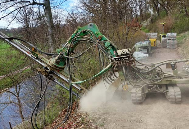
The TITAN micropiles were installed with small equipment near preserved vegetation.
